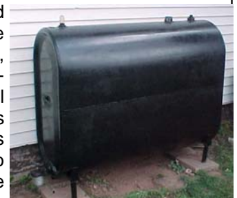
Domestic Fuel Oil Tank
